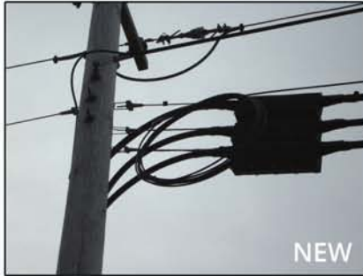
Fiber Optic Connection
