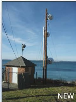
1GbE true throughput licensed Microwave Link at Shore Point with five-nines availability
